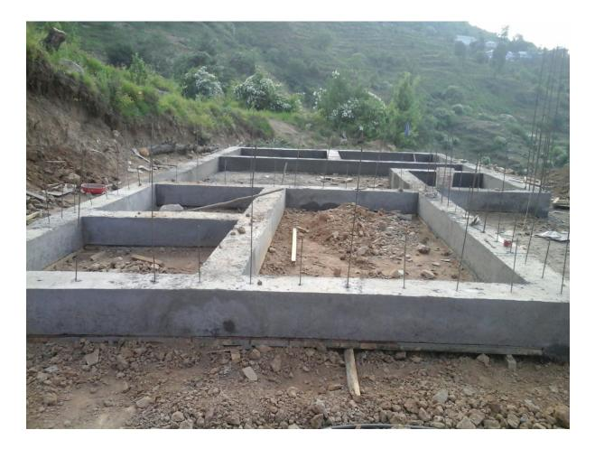
Walls are strong due to 150 mm concrete Core, designed as per IS456:2000 and IS:875 for earthquake resistant design . Concrete poured is of grade M-20 inside 50 mm hollow panels of EPS formwork on both sides.
