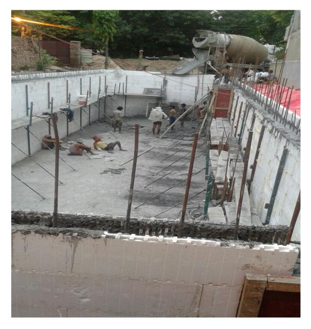
**Reinforcement** Steel bars of dimensions conforming to structural design as per IS456.
