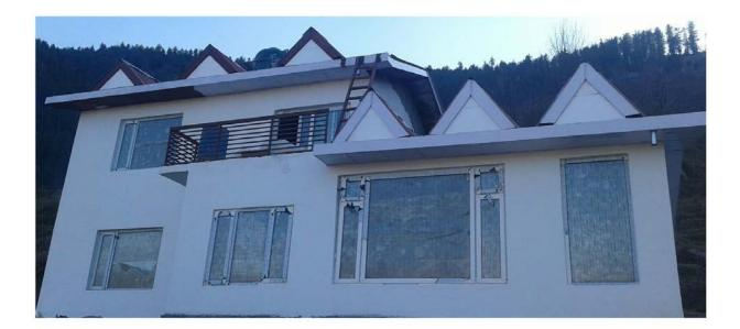
Typically, the main finish is a render or render-equivalent covering or paint. Any additional cladding can be added to the ICF walls subject to making appropriate supports for it, although many sheet finishes, such as plasterboard, can be glued directly to the surface of the formwork.
